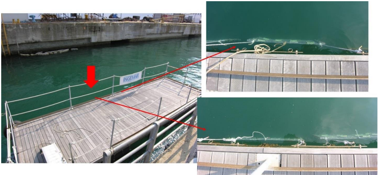
Figure 86 Immersion of the frames on the side of the raft at the SMS of IAS-CNR.
