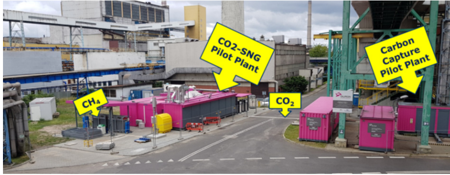
Figure 3.1: Power-to-gas demonstrator at the Łaziska power plant.
