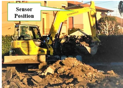
Fig. 19. Testing Inclinometer in Excavator
