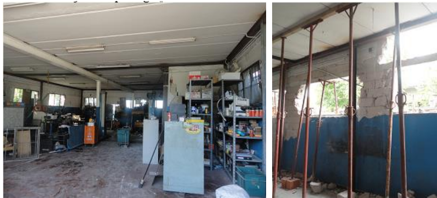
Figure 8 (a) Internal view of groundfloor and (b) detail of diagonal cracks in masonry piers between adjacent openings.
