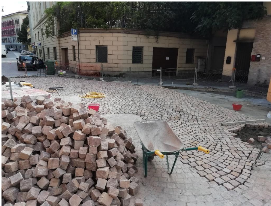
75 76 77 78 79 80 Figure 1 - Construction of a stone pavement in urban context
