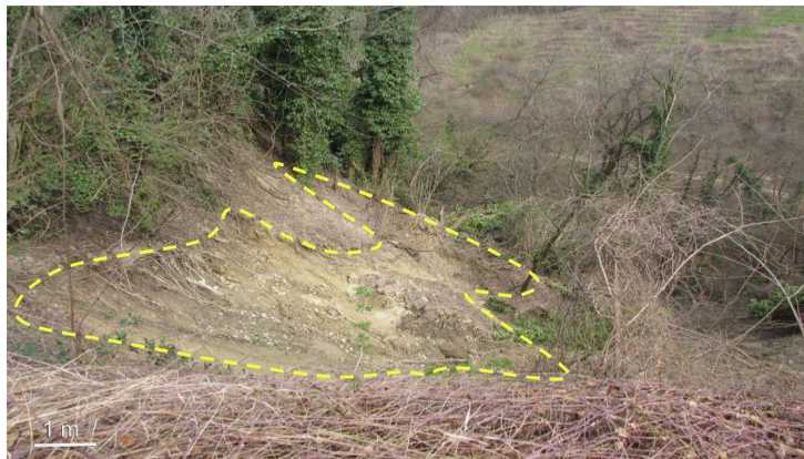
Figure 3.4: The 2014 landslide (location and size are reported in Fig. 3.2)
