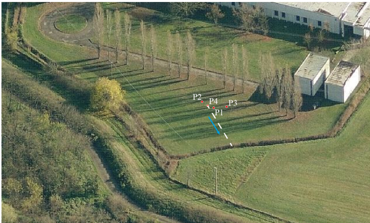
Figure 6.3: View of the well field.
