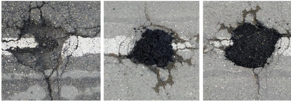
Figure 1. Patching a pothole with CPM
