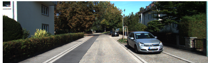
(a) curbs with too low elevation
