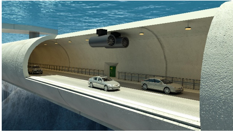
Figure 2.31. Conceptual design of the “Archimedes Bridge” [187].
