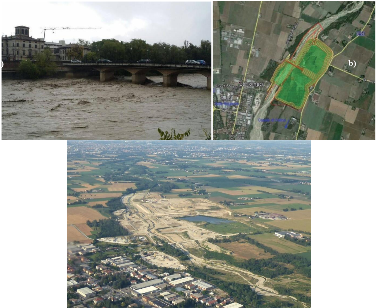
Figure 5.1 a) Flooding due to heavy rainfall on October 13, 2014, which also affected road infrastructures and settlements closest to the engraved Baganza River. b) Cassa di espansione sul torrente Baganza project capable of making the Parma city safe. c) Closer look of the cassa di espansione work under progress July 2023.
