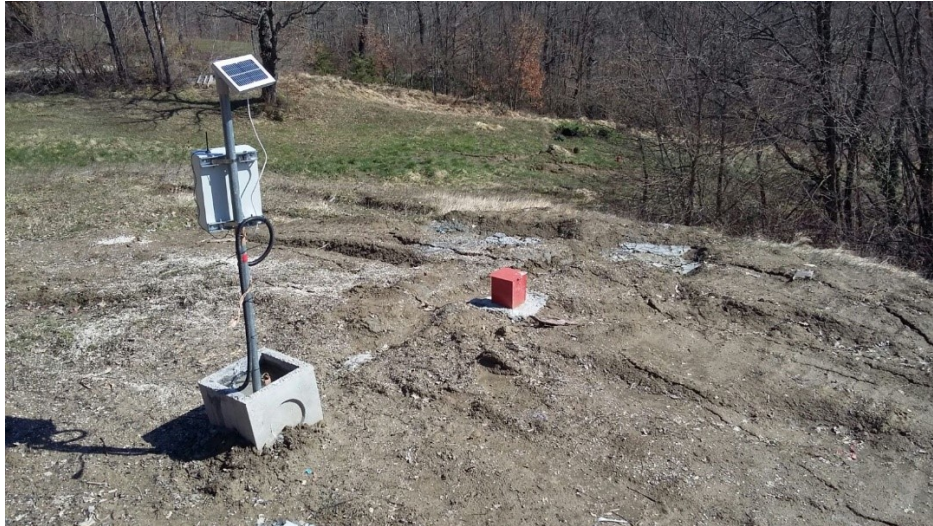
Figure 51. Installation site of Vertical Array DT0014
