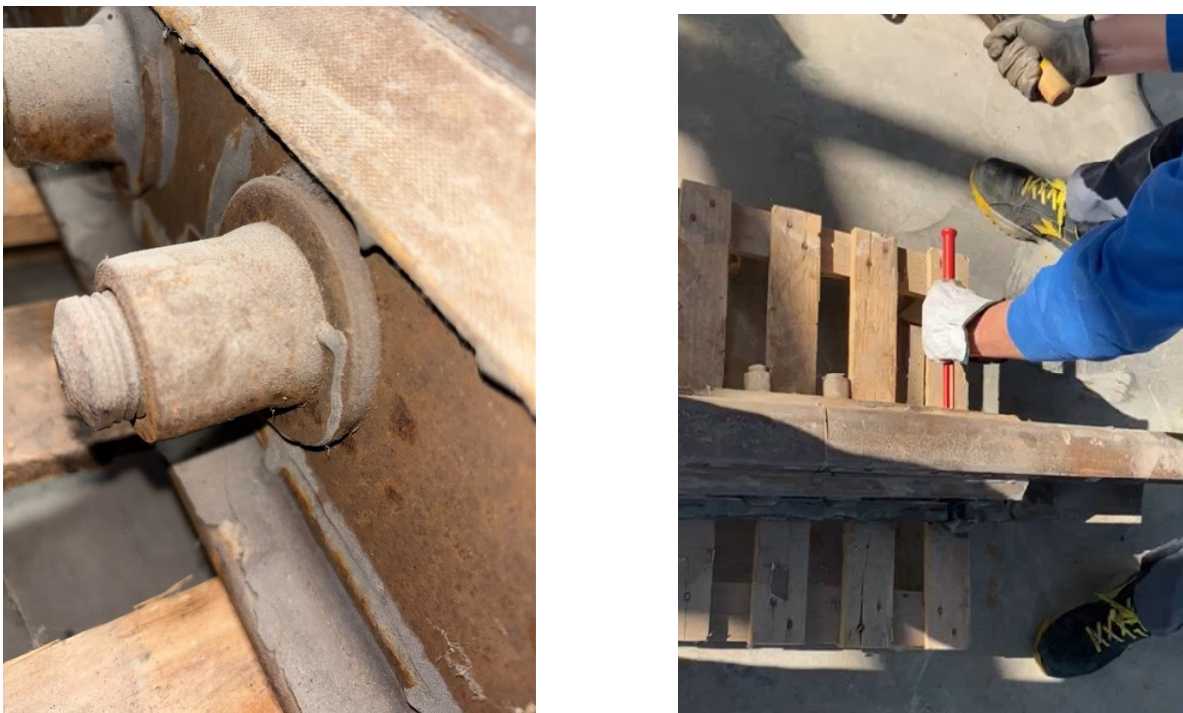
Figure 74. Original bolt anti-rotation collars and bolts extraction
