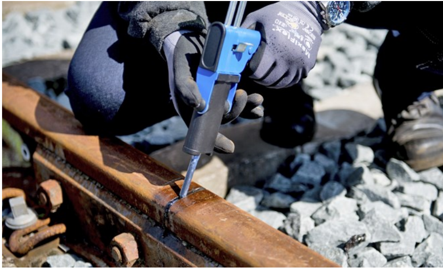
Figure 27. IRJ's end post repair operation
