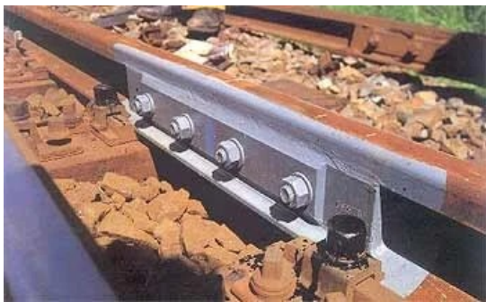
Figure 15. IRJ with four and six bolts
