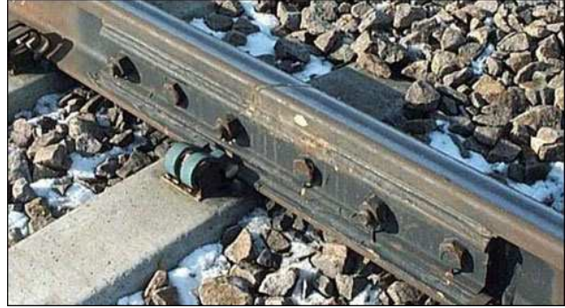
Figure 17. Suspended and supported IRJ
