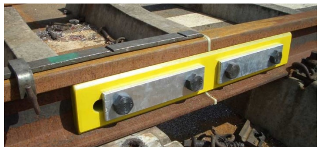
Figure 16. Glued and non-glued IRJs
