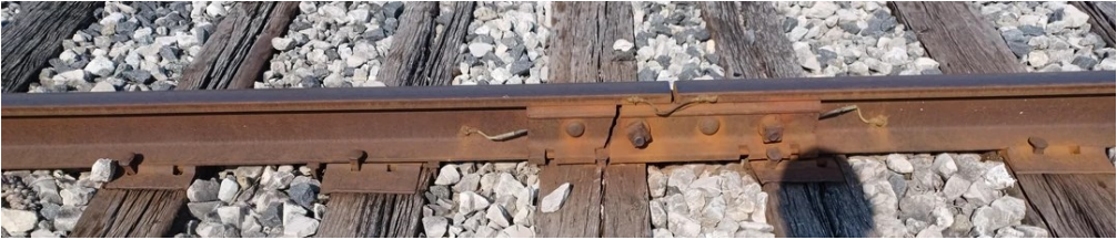
Figure 26. Cracked fishplate
