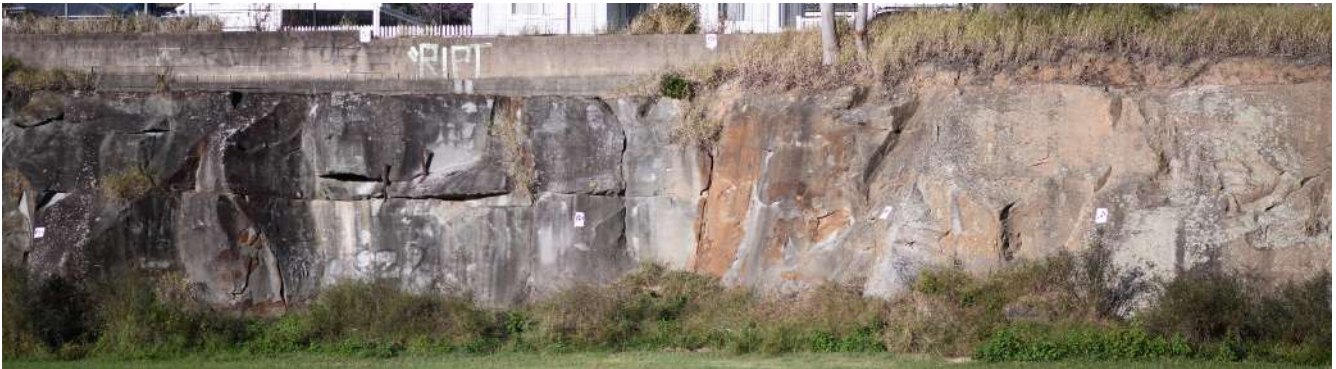
Figure 6. Overview of the rock face at Pilkington Reserve (Site 1).
