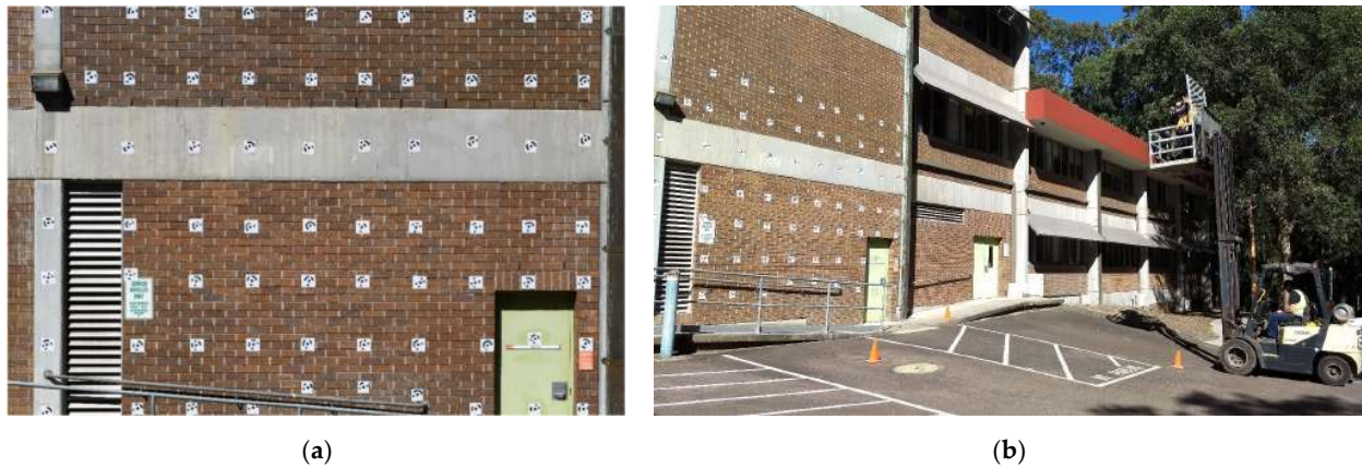
Figure 2. Full-field (FF) calibration setup: (a) Front view of the coded targets; (b) image acquisition of the target field using a forklift with a safety cage.
