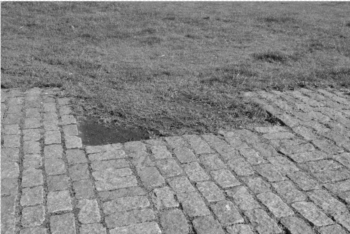
Figure I.16 | A detail of the new permeable pavement and vegetation introduced with the soil desealing intervention in Clausplein in Eindhoven, the Netherlands. Source: photo taken by the author (2023).
