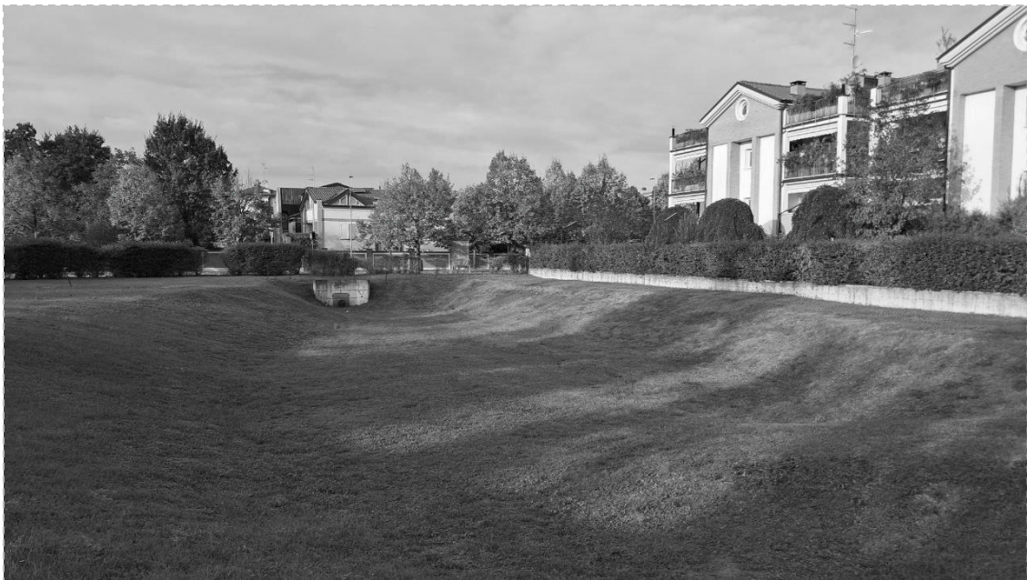
Figure III.32 | An example of a detention pond located in the southern neighbourhoods of Parma. Source: photo taken by the author (2024).
