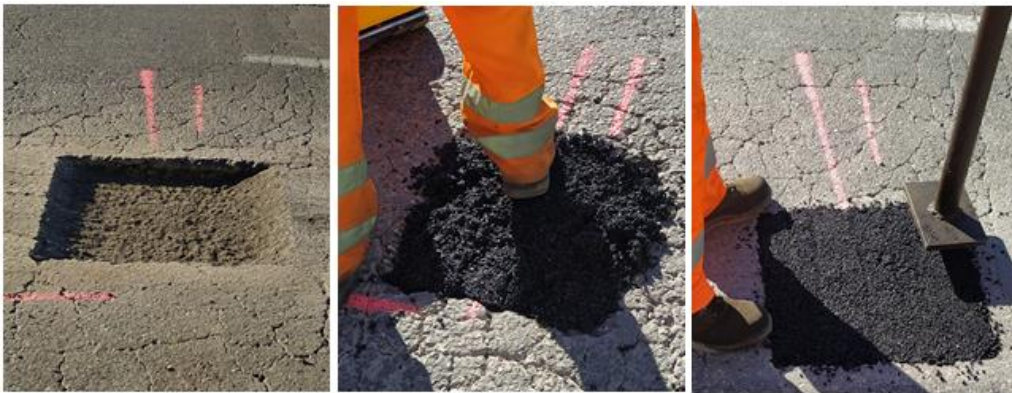
Figure 1.2. Using a CMPM to patch a pothole
