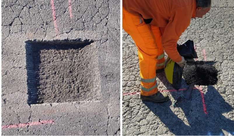
Figure 6.4 Pouring the material into the clean potholes
