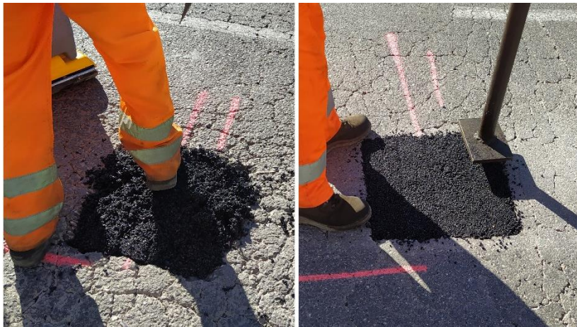
Figure 6.5 Using feet and hand tamper to compact the patching materials
