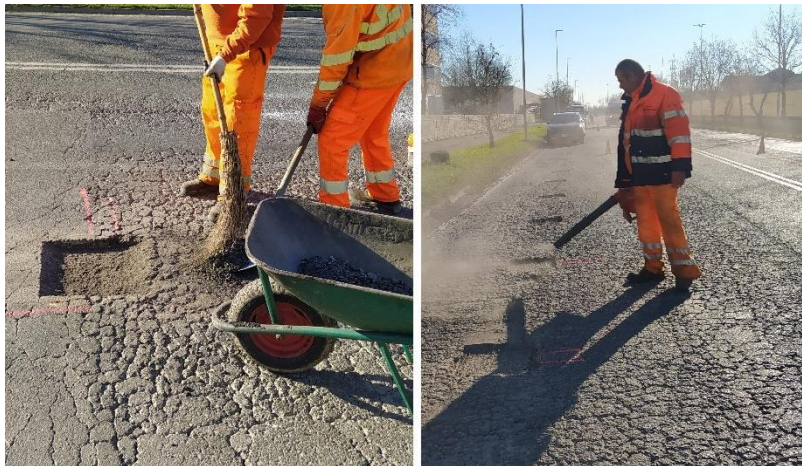
Figure 6.3 Cleaning the potholes by removing dusts and debris
