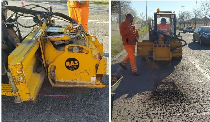
Figure 6.2 Creating square potholes using an asphalt milling machine
