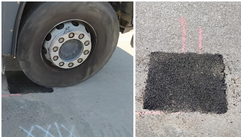
Figure 6.7 Passing the truck for final compaction
