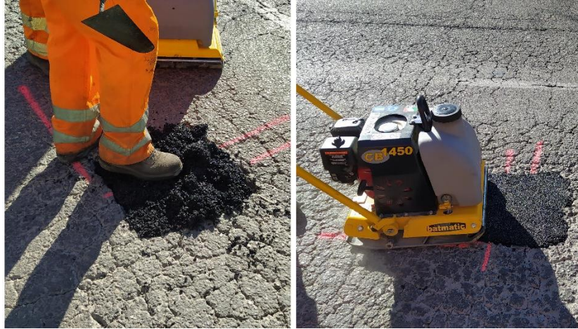
Figure 6.6 Using feet and a vibratory forward plate compactor to compact the patch
