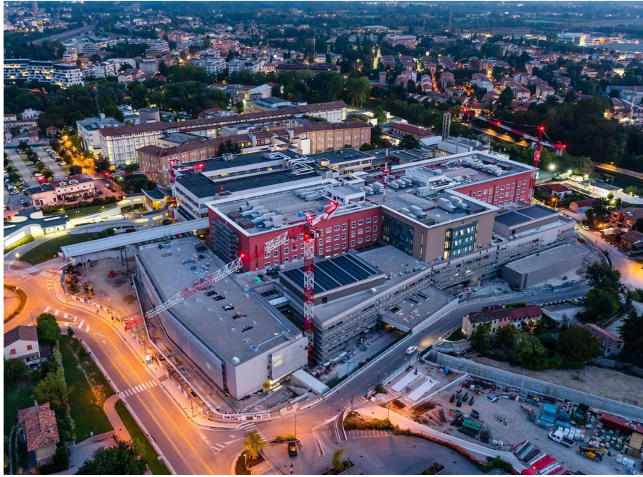
FIGURE 4.4: Ca'Foncello Hospital in Treviso
