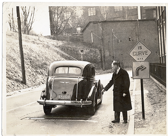
Figure 12: Charles Adler Jr. showing one of his safety systems, which triggers a light when a car pass over a sound detector
