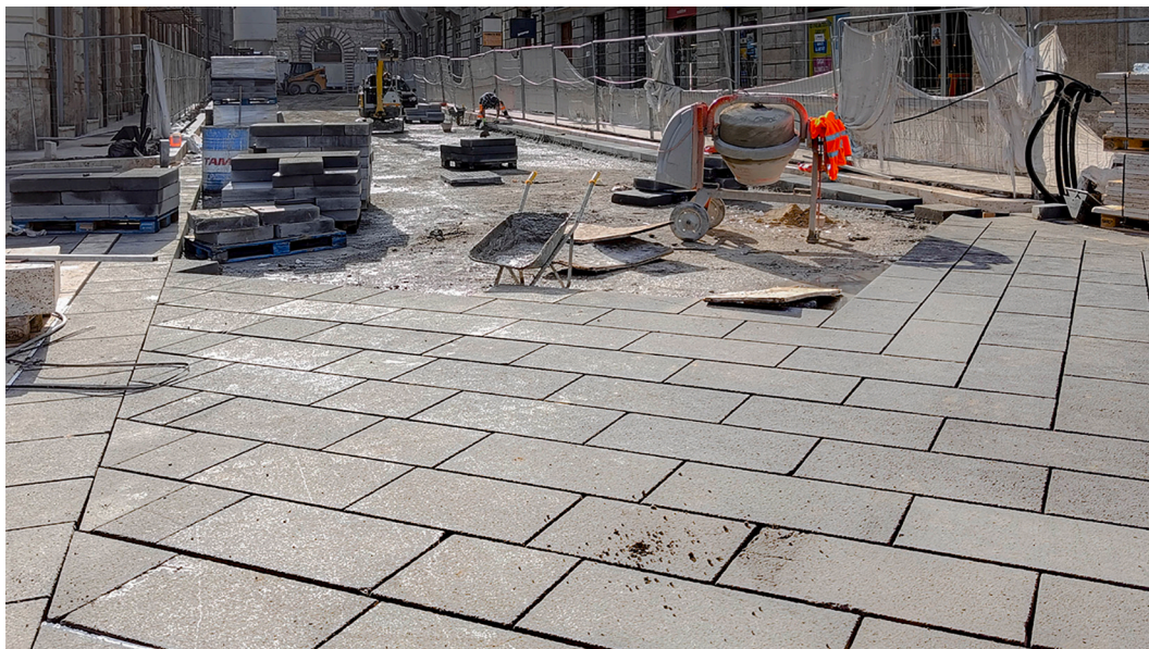
Fig. 1. Construction of a street pavement using igneous stone blocks.
