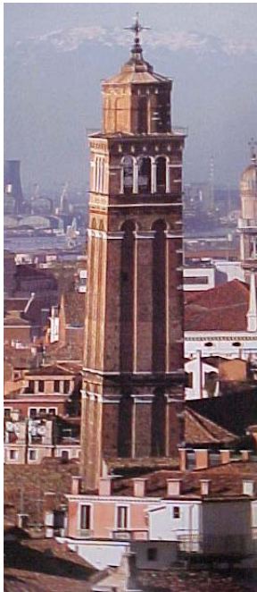
Figure 1.10. Picture of the tower.
