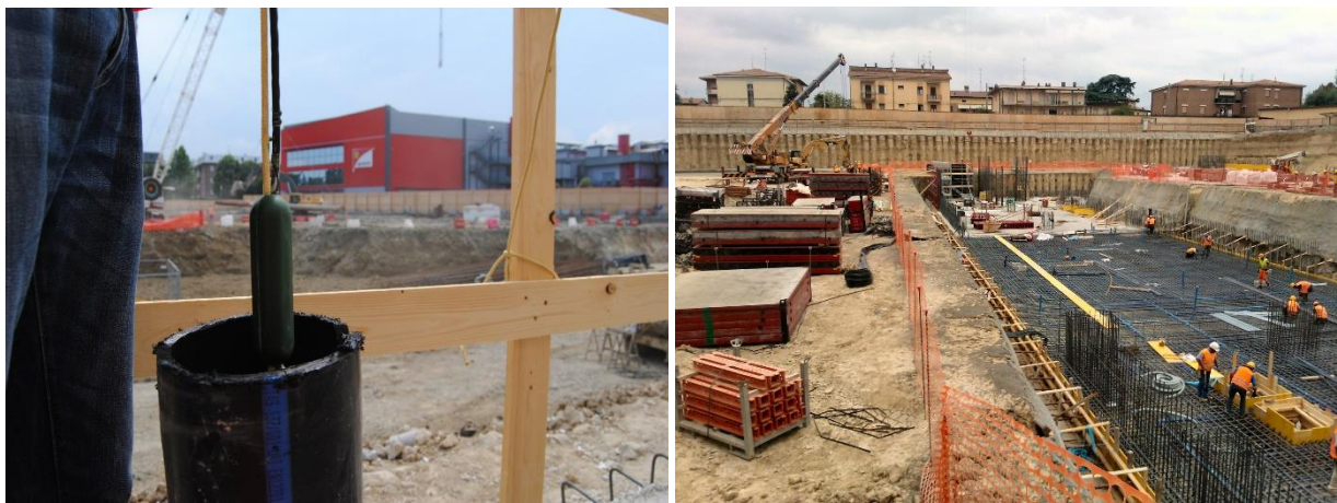
Fig. 5.1: Construction site of Ferrari GeS
