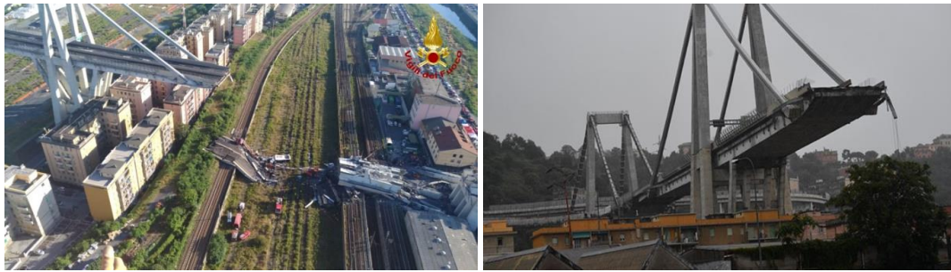
Fig. 1.9: Collapse of the Morandi Bridge in Genova (14 th August 2018)
