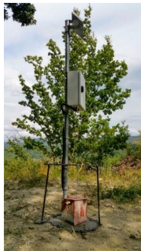
Fig. 5.30: MUMS DT0014 after installation on site
