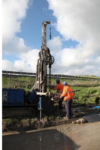
Fig. 5.12: Installation of MUMS monitoring system
