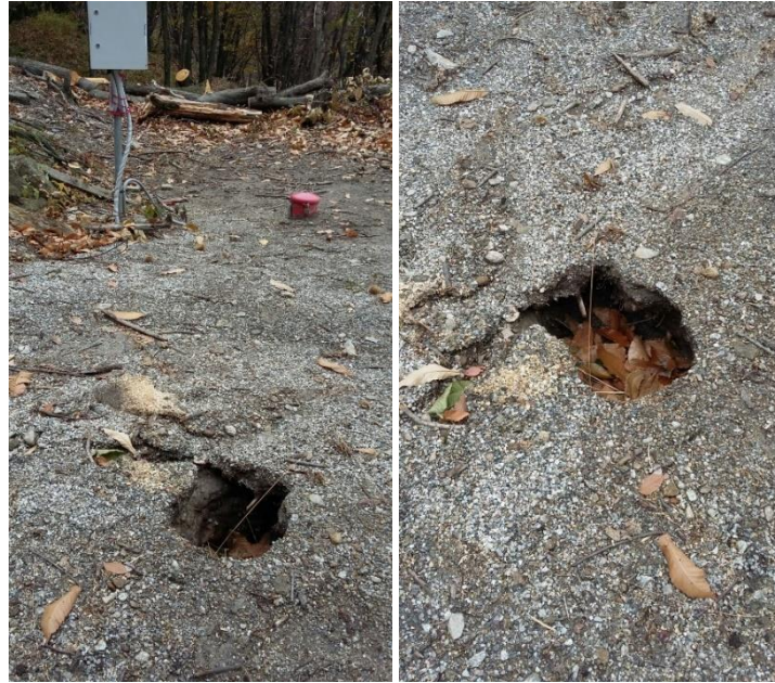
Fig. 3.20: Site inspection at Baveno, after the event occurred on December 2017
