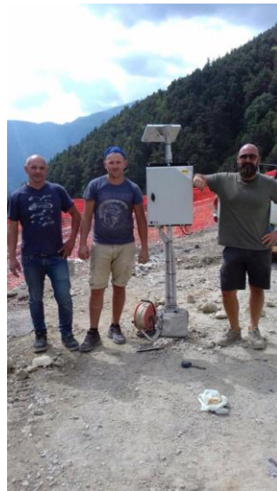
Fig. 5.45: Installation of DT0080 and DT0081 MUMS Vertical Arrays
