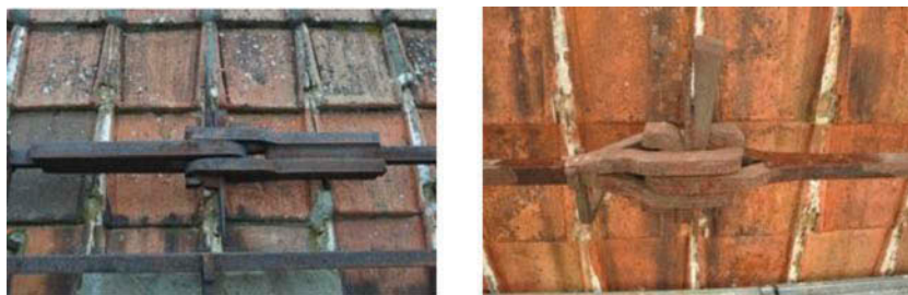
Figure 24. Two different junction systems present on the dome, belonging to the two different period: (a) 1570 and (b) 1620.
