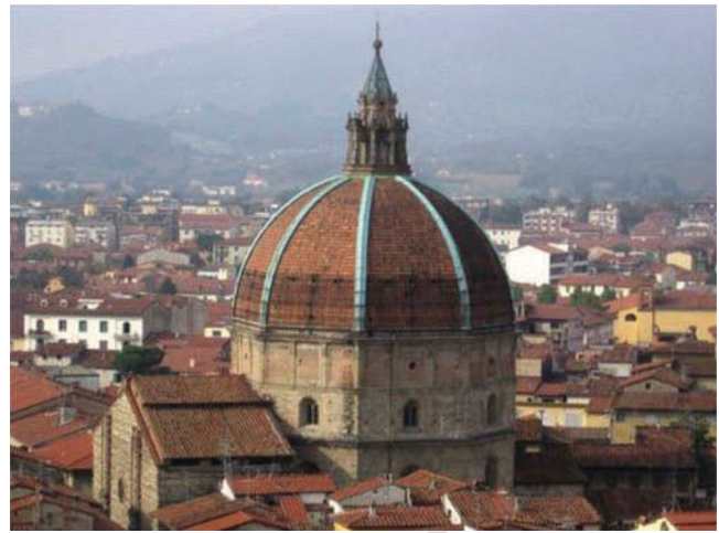
Figure 17. The dome of Madonna dell’Umiltà in Pistoia and its outer iron chains, clearly visible.
